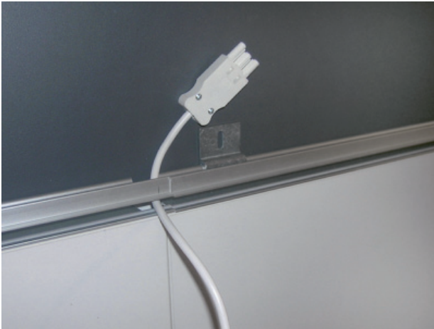
3) Position connecting cable.
